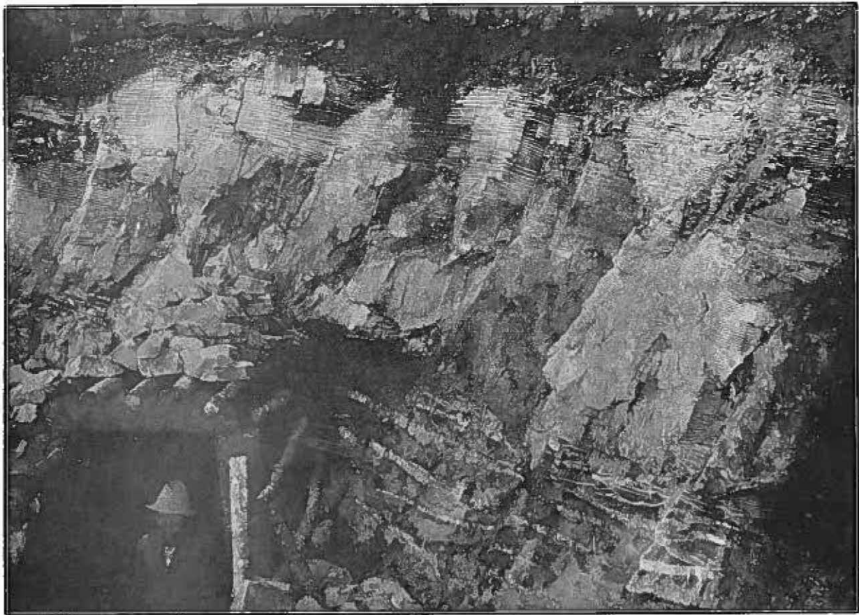
PLATE XII.— Typical Section across the Ribbon Line of the New Amianthus Mine near Kaapsche Hoop (Barberton District) to show the characteristic upper portion with many parallel chrysotile seams, and the lower portion with a few, more widely spaced, thick seams.
